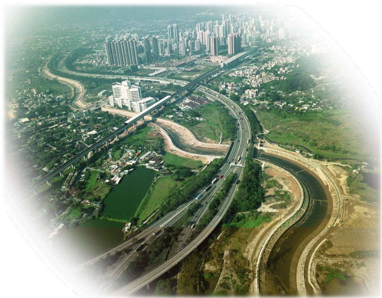
Yuen Long Bypass Floodway
